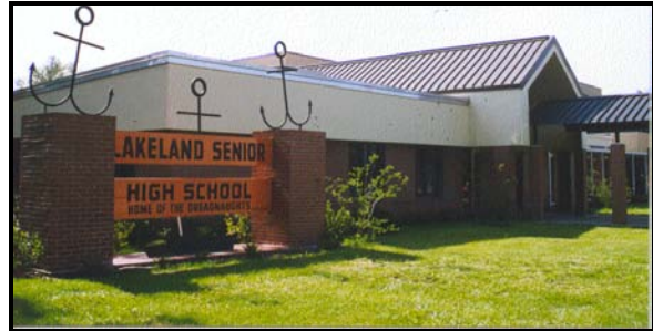
Addition to Administration Office
